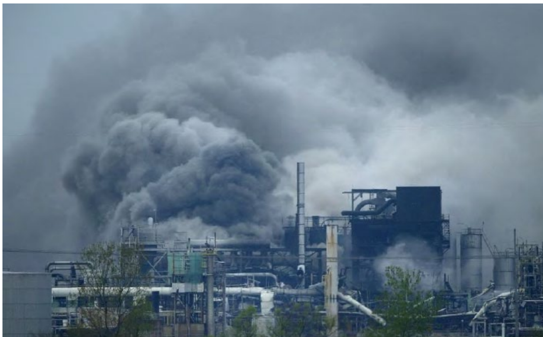
Vinyl Chloride Explosion, Formosa Plastics, Illioopolis, April 23, 2004.
