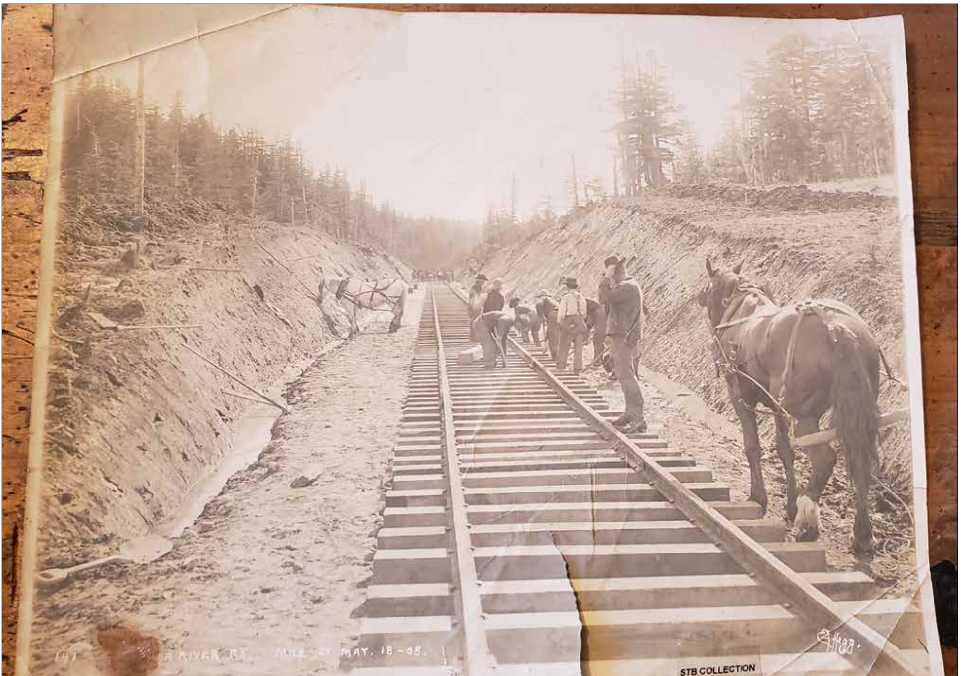
Thanks to history buff Shawn Beiswenger for sharing this image from his collection. This photo, dated from 1908, shows workers constructing the Copper River Railroad.
