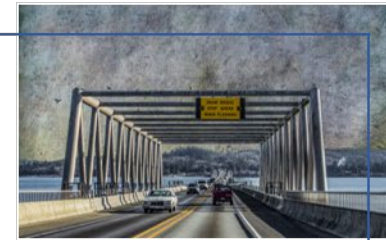
Hood Canal Bridge
