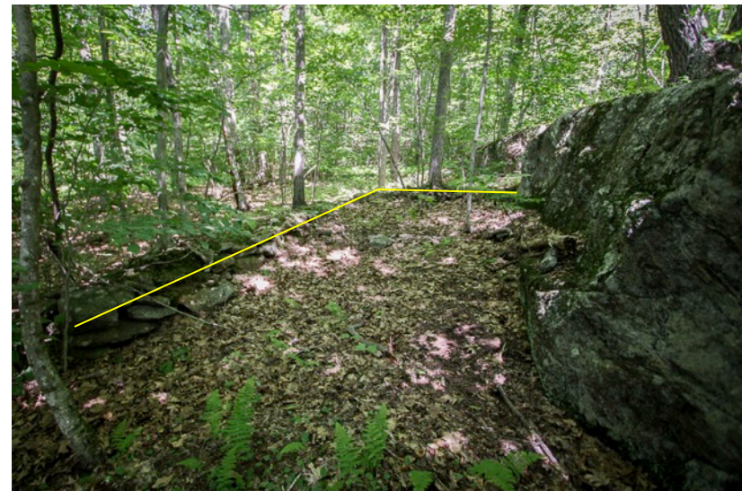
BARN FOUNDATION uses the bedrock ledge on the right and stacked stones on left and far end (yellow lines).
