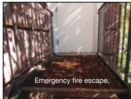
Emergency egress door. Note sloping landing.
