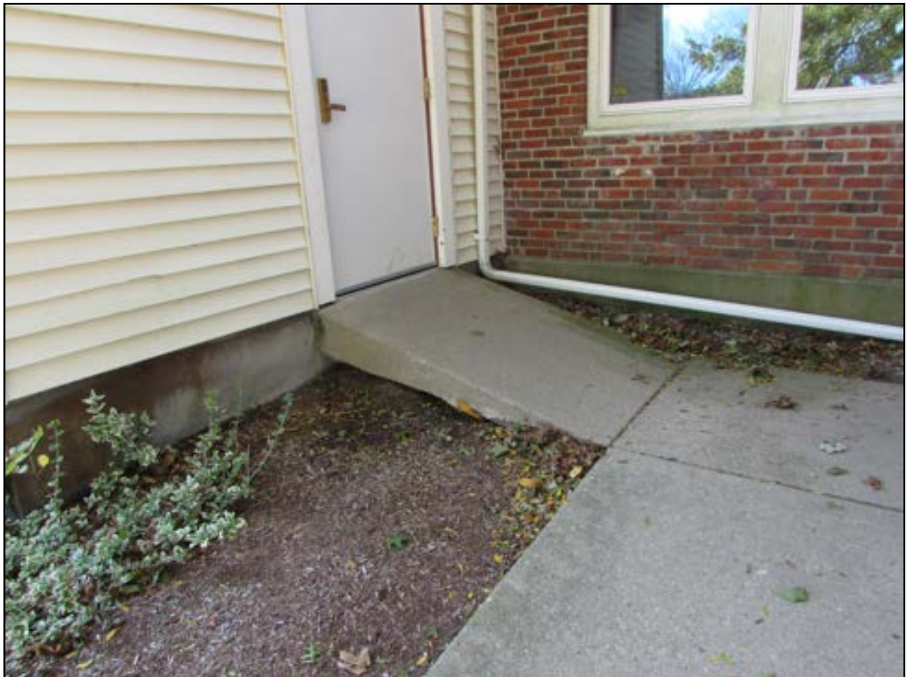
Service Entrance landing outside Receiving and Staff Work Room areas.
