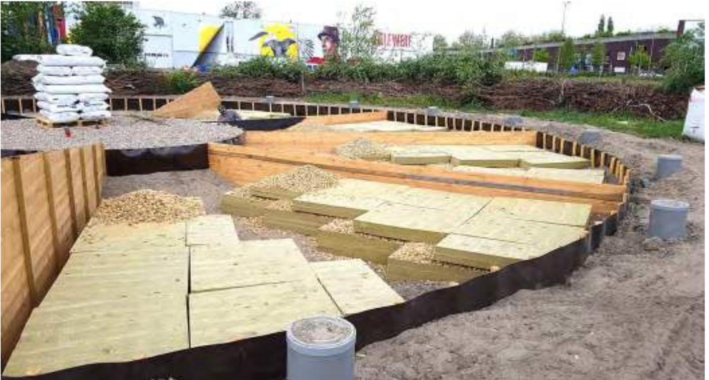
Placing soil in-between the Lapinus and gravel layer for infiltration and ventilation
