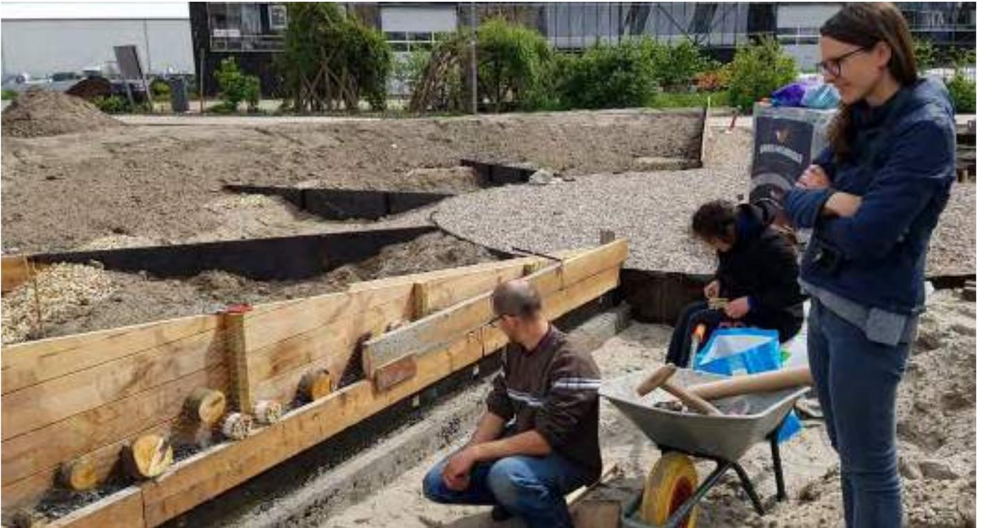
Inserting wood, bamboo and balloons to create voids for organic matter
