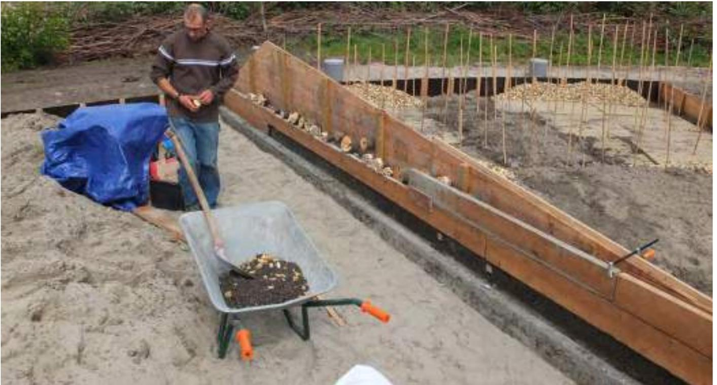
Compacting the clean sand as if it were a road foundation layer
