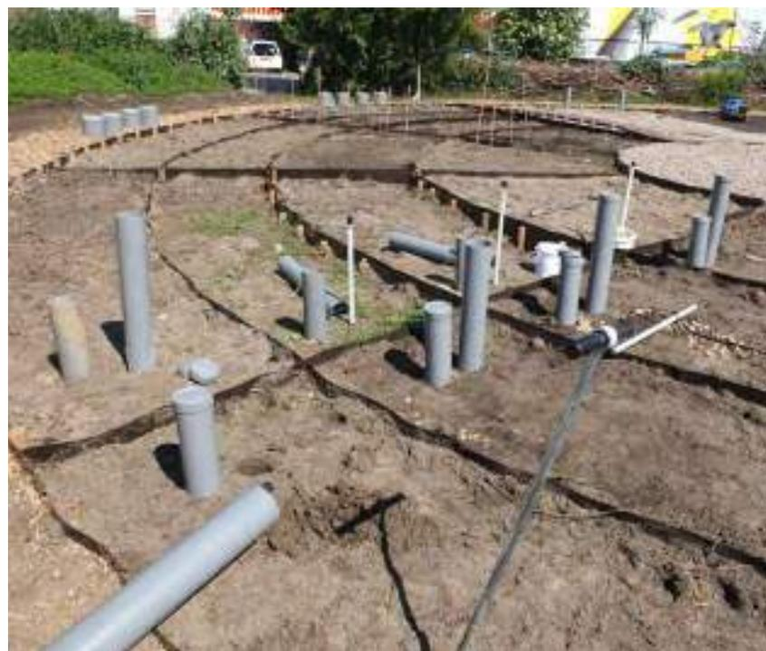
*Installation of the hydrological monitoring pipes and the digital water loggers*
