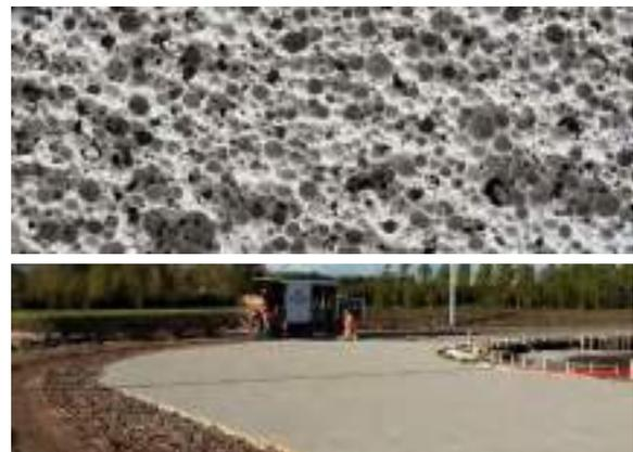
*Porous concrete is a special type of concrete with a high porosity that allows water from precipitation to flow through it. Thereby it reduces runoff/drainage and allows groundwater to recharge. It is mainly used in parking areas with light traffic, residential streets, pedestrian paths and bike trails.*
