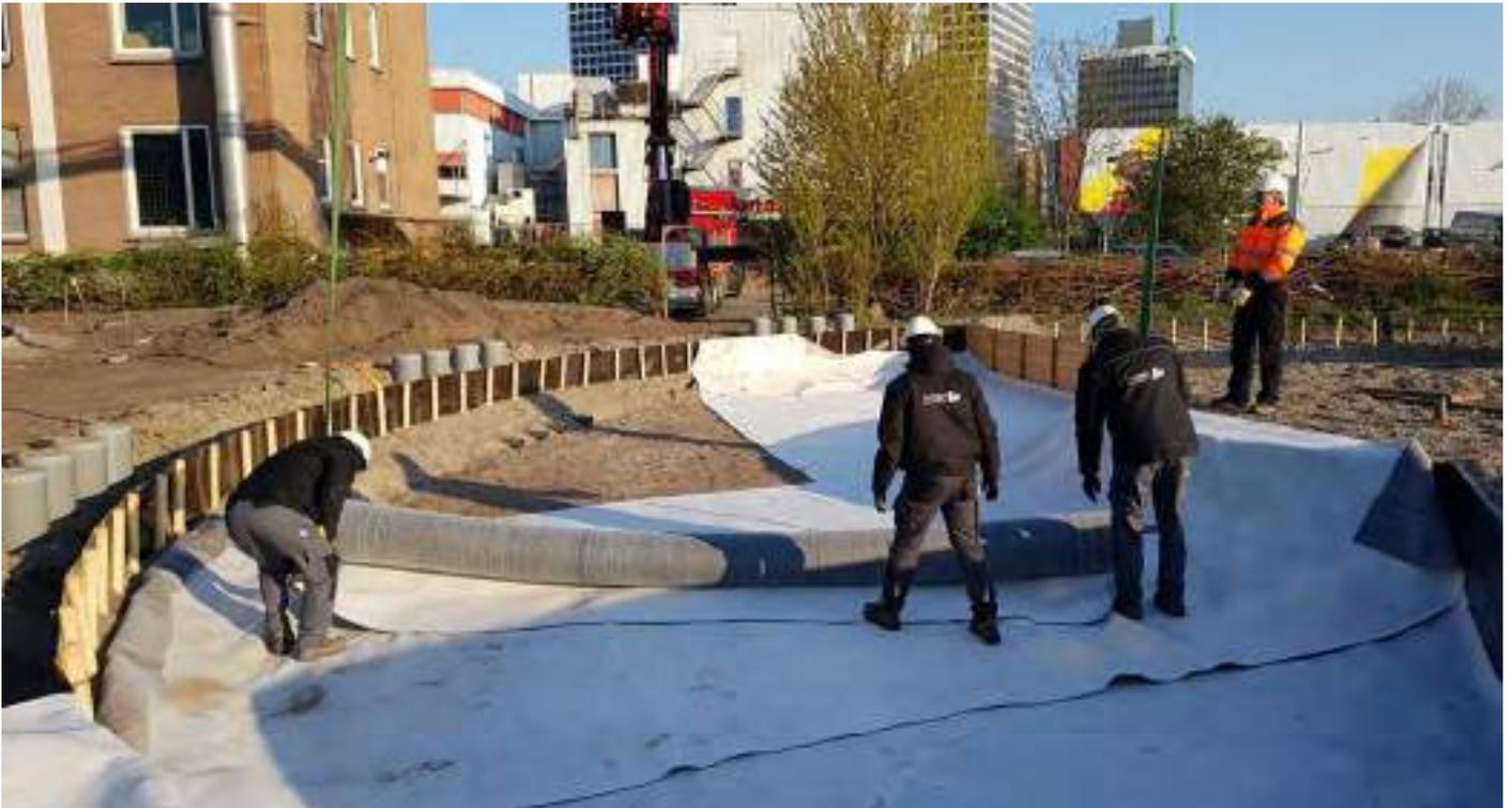
Separating various soils to allow monitoring - installing root shields, drainage pipes and a gravel layer
