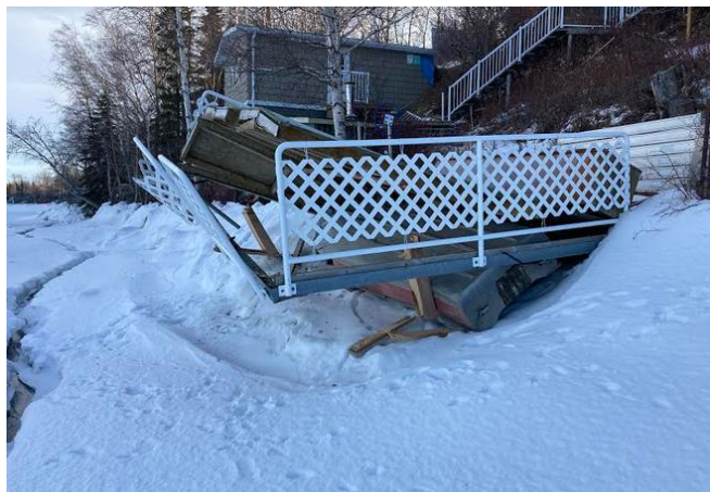
Photo 1: Ice heaves damaging shoreline infrastructure
