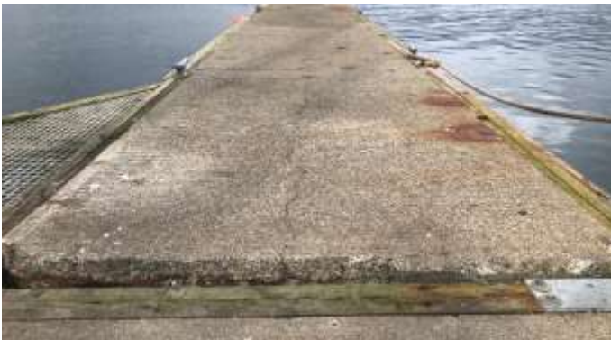
Figure 4-5: Deteriorated Floats
