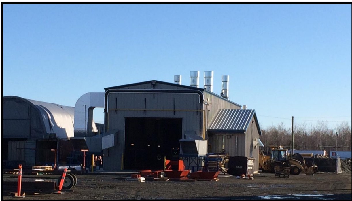
FIGURE 4: NEW MFE MANUFACTURING BUILDING, CITY OF MIRAMICHI
