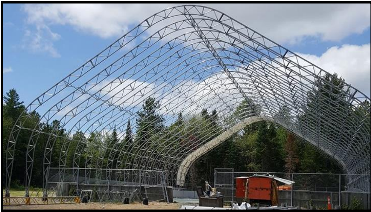
FIGURE 9: MULTIPURPOSE AREA ROOF ADDITION, RURAL COMMUNITY OF UPPER MIRAMICH
