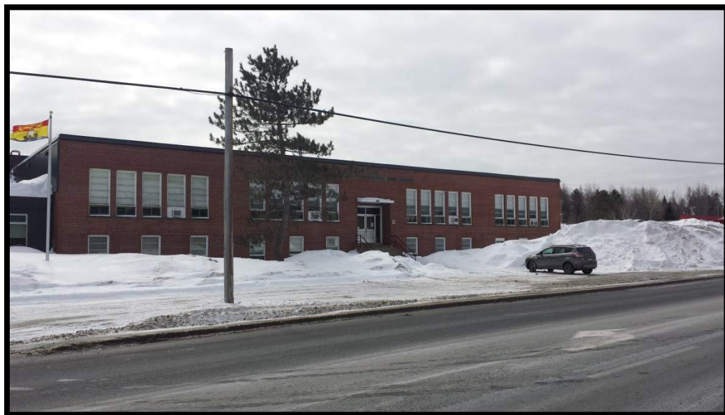
FIGURE 14: DOAKTOWN ELEMENTARY SCHOOL, VILLAGE OF DOAKTOWN
