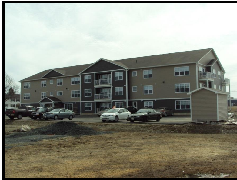
FIGURE 9: MARTELL 23-UNIT APARTMENT BUILDING, CITY OF MIRAMICHI
