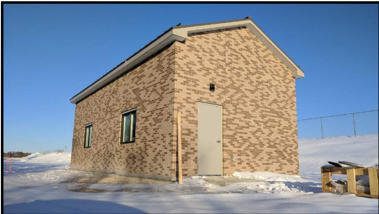
FIGURE 6: NEW UV WASTE WATER TREATMENT FACILITY, CITY OF MIRAMICHI
