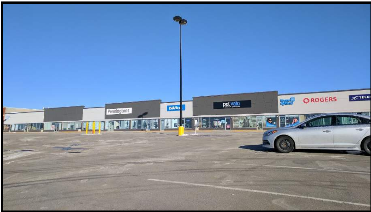
FIGURE 9: BRIDGEVIEW PLAZA FAÇADE IMPROVEMENTS, CITY OF MIRAMICHI
