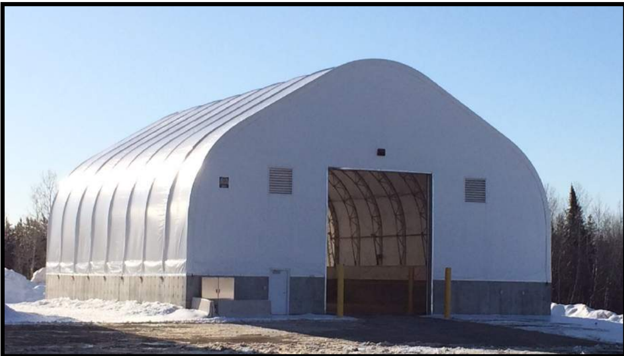
FIGURE 8: NEW SALT STORAGE FACILITY, RENOUS
