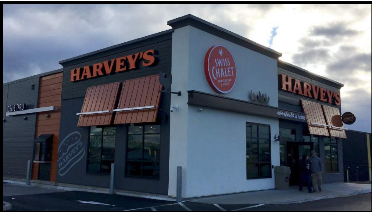
FIGURE 4: NEW SWISS CHALET / HARVEY'S RESTAURANT, CITY OF MIRAMICHI
