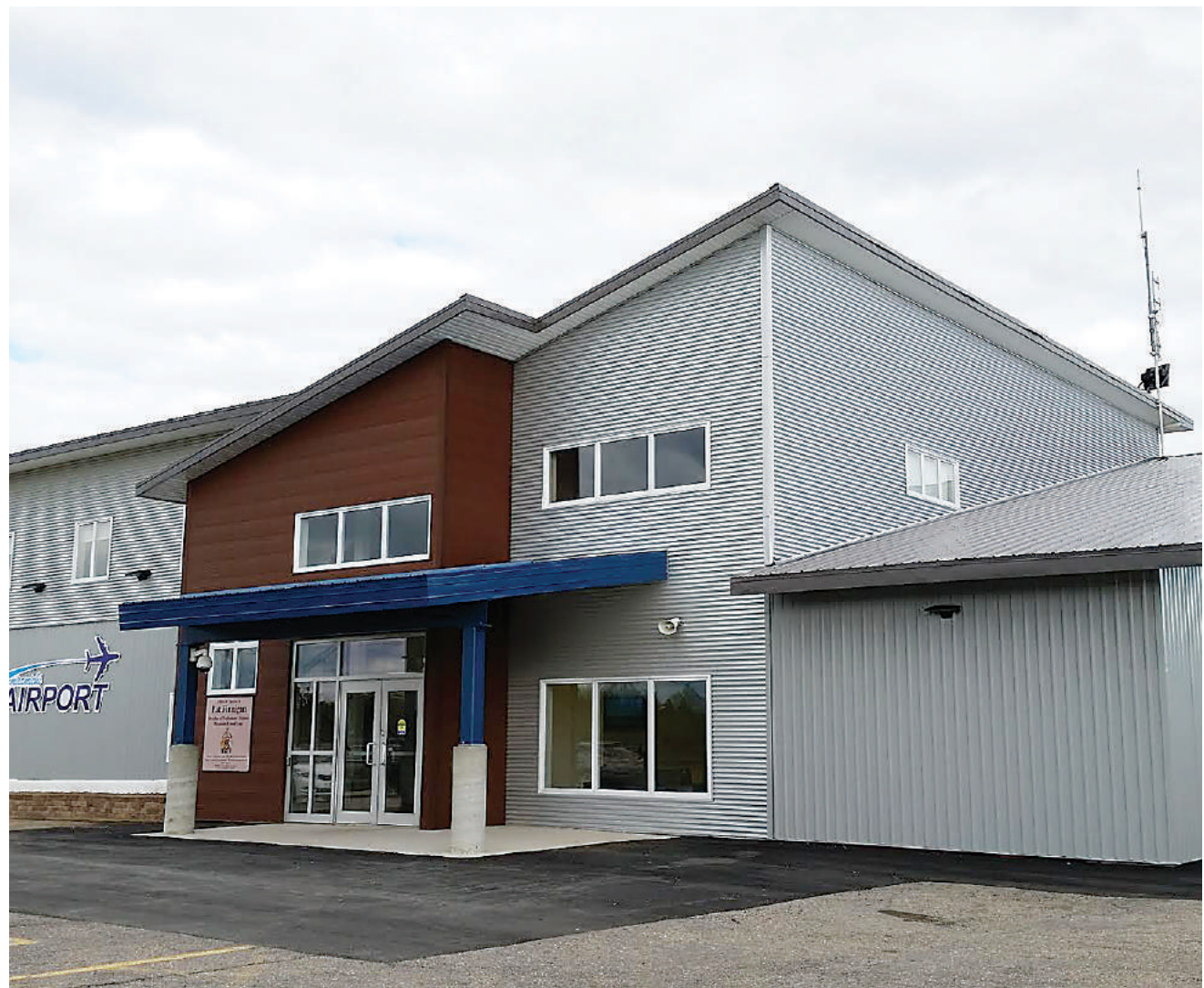
A look at the exterior of the new $1.5 million Miramichi Airport terminal. Airport officials are asking for financial contributions from the area's municipalities to help the facility with its long-term growth agenda. PHOTO: KRIS MCDAVID/MIRAMICHI LEADER
