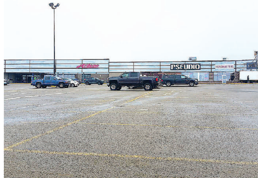
A look at the new facade of the redesigned Northumberland Square mall in Miramichi. The developer, Rio Plaza Properties Inc., were presented with the first ever Silver Shingle award for excellence in development at a recent Greater Miramichi Regional Service Commission meeting. PHOTO: KRIS MCDAVID/MIRAMICHI LEADER
