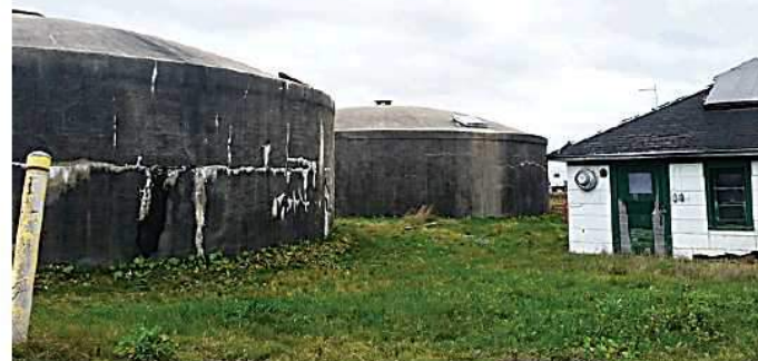
All three of these water outdated waterworks buildings on the former CFB Chatham property will be demolished in the coming weeks, along with a number of others in the city, as it moves ahead with a modernization of its systems.
