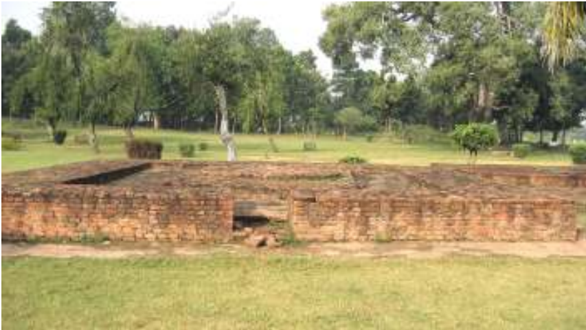
Plate 39: On entering the ancient ruins after the Ananda Bodhi tree, the first shrine on the left is believed to mark the very spot where the original Kosambi kuti, built by Anathapindika for the personal use of the Buddha, once stood. Just across it is a raised brick platform to mark the site of the cankama , where the Buddha practiced walking meditation.
