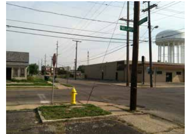
Figure 1 – Overhead Power Lines Obstructing View. Photo: Laura Dodd.
