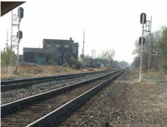
Figure 8 – The railroad across Walnut Street. Photo: Kyle Herrera.
