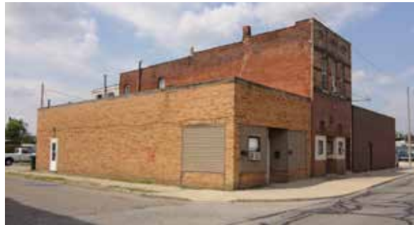
Figure 5 - A vacant structure along Walnut Street. Photo: Mandy Dyer.
