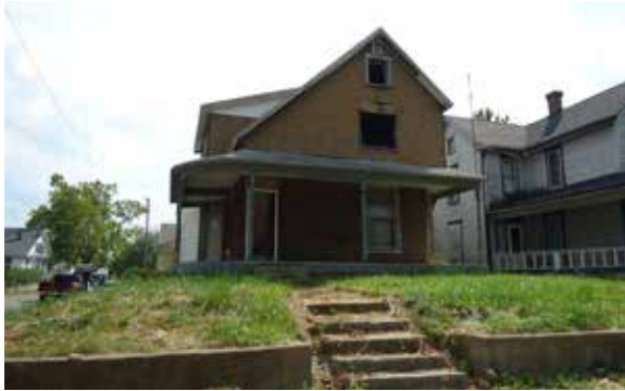
Figure 2 – A house that was recently torn down. Photo: Giang Tran.
