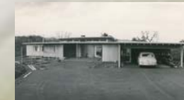
As in Vermont, Wallace did much of the new house's carpentry and landscaping himself.
