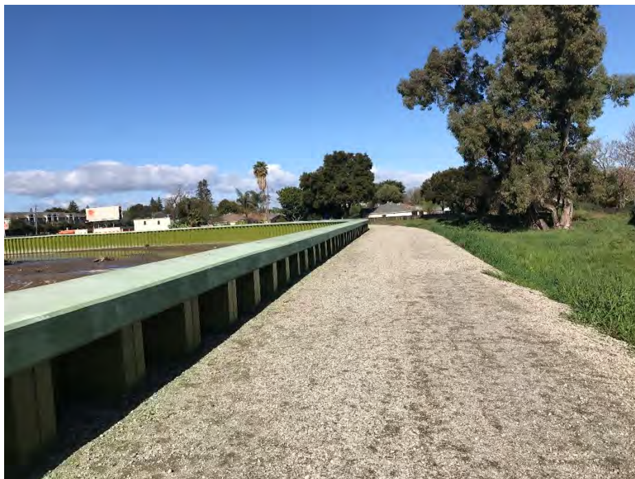
Figure 2-9. Example Sheet Pile Floodwall
