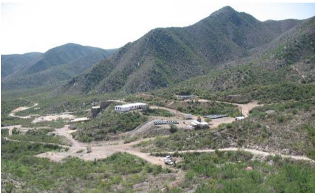
Figure 6: View looking SE of the exploration buildings, logging and core storage areas (photo taken in 2012).
