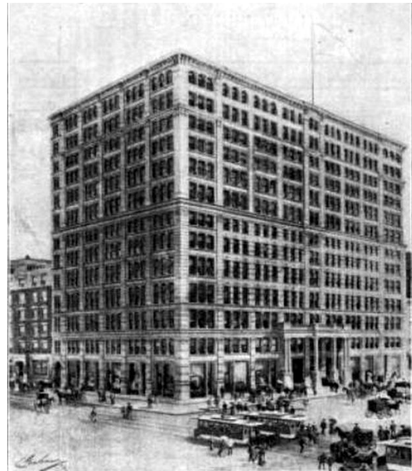
The American Lithographic Building is a 13 story steel-frame structure built by Ford, Bacon & Davis in 1895. American Lithographic Co. remained in this building until 1930 though the building itself still remains.
