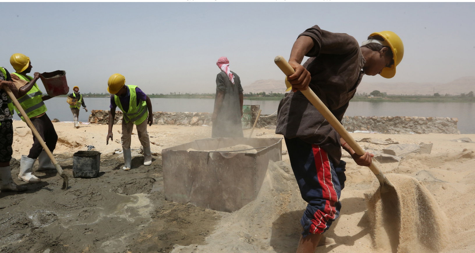
Egypt Emergency Labor Intensive project - Luxor, Epyt - World Bank Photo Collection
