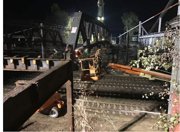
Figure 1 : Lloyd Street Bridge Removal
