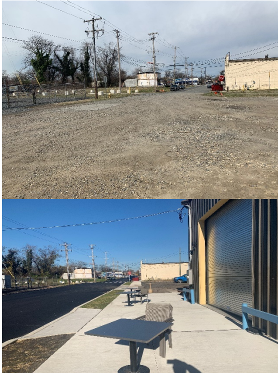
Figure 2: Before and After Photos of Engle Street Reconstruction
