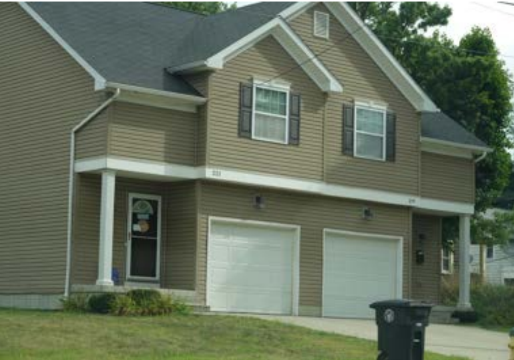
Duplex in Summit Lake built by the City of Akron using Neighborhood Stabilization Program (NSP) funds. Building was purchased by AMHA and is used as scattered site public housing.
