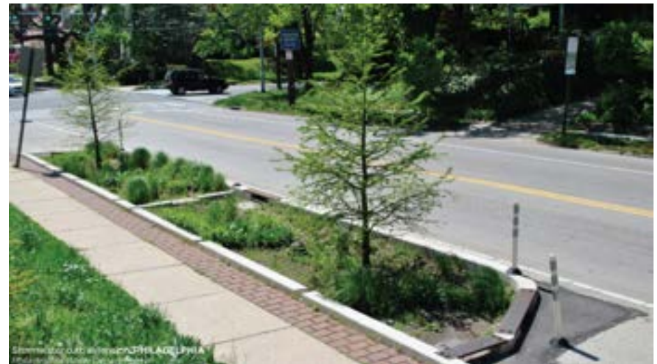
Example of stormwater curb extension
