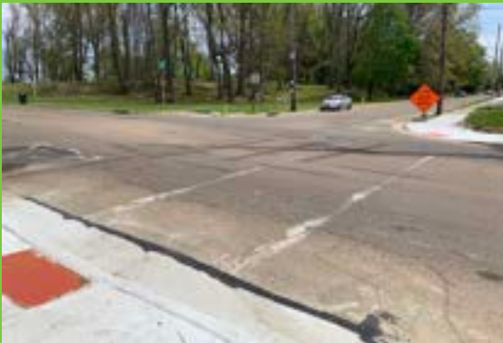
Curb ramps at Long Street and Lakeshore Boulevard.
