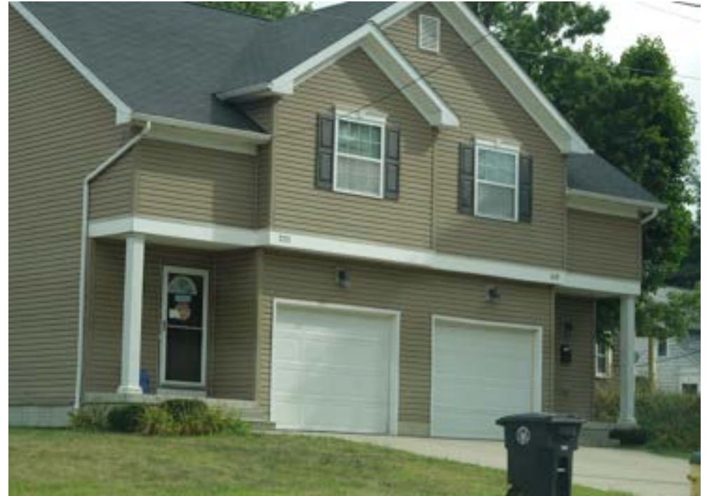
Duplex in Summit Lake built by the City of Akron using Neighborhood Stabilization Program (NSP) funds. The building was purchased by AMHA and is used as scattered site public housing.
