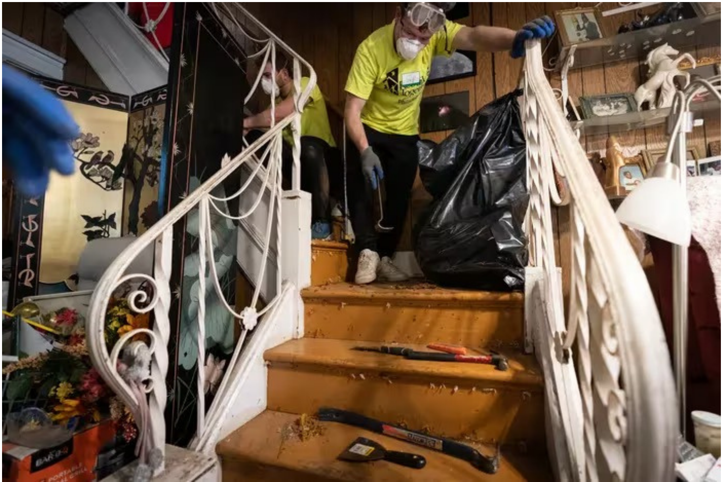
Volunteer Guy McKhann pulls nails from the steps after removing the carpet in the home of Deborah Ryles. Jessica Griffin / Staff Photographer
