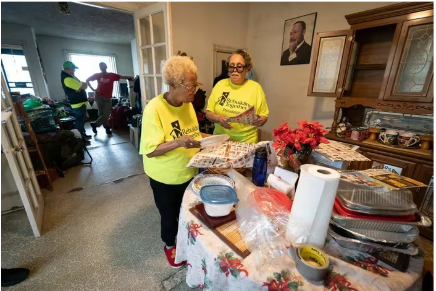
Jane Stevens (left) and Linda Smith box up dishes in their West Philadelphia dining room to make space for the installation of new flooring.
