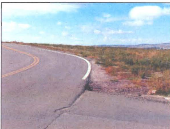
No sidewalks were present along portions of South Pine Drive.
