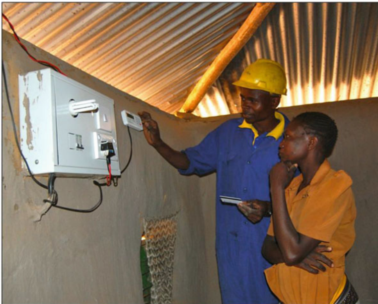
Fig. 5.5 Umeme Rahisi ready-board solution designed by Power Technics
