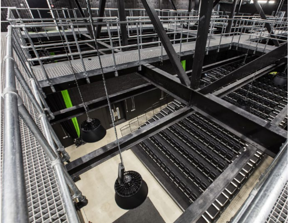
Above: Photograph of the film studio gantry and truss structure
