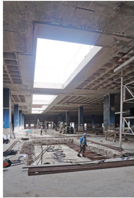
Above: Large voids were cut into the building to bring light in the heart of the space.
