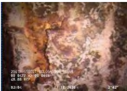
Photo 6-1 216 th Street CCTV View
