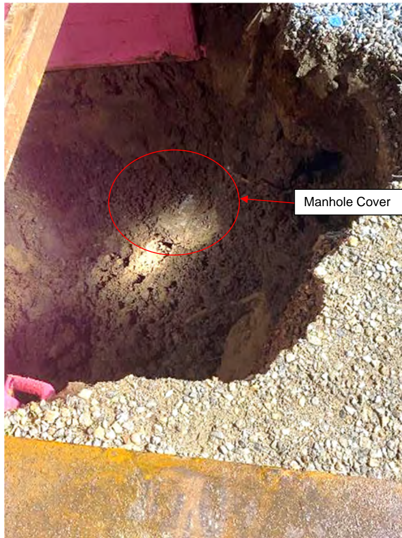
Photo 3-6 Excavation in the Failure Area
