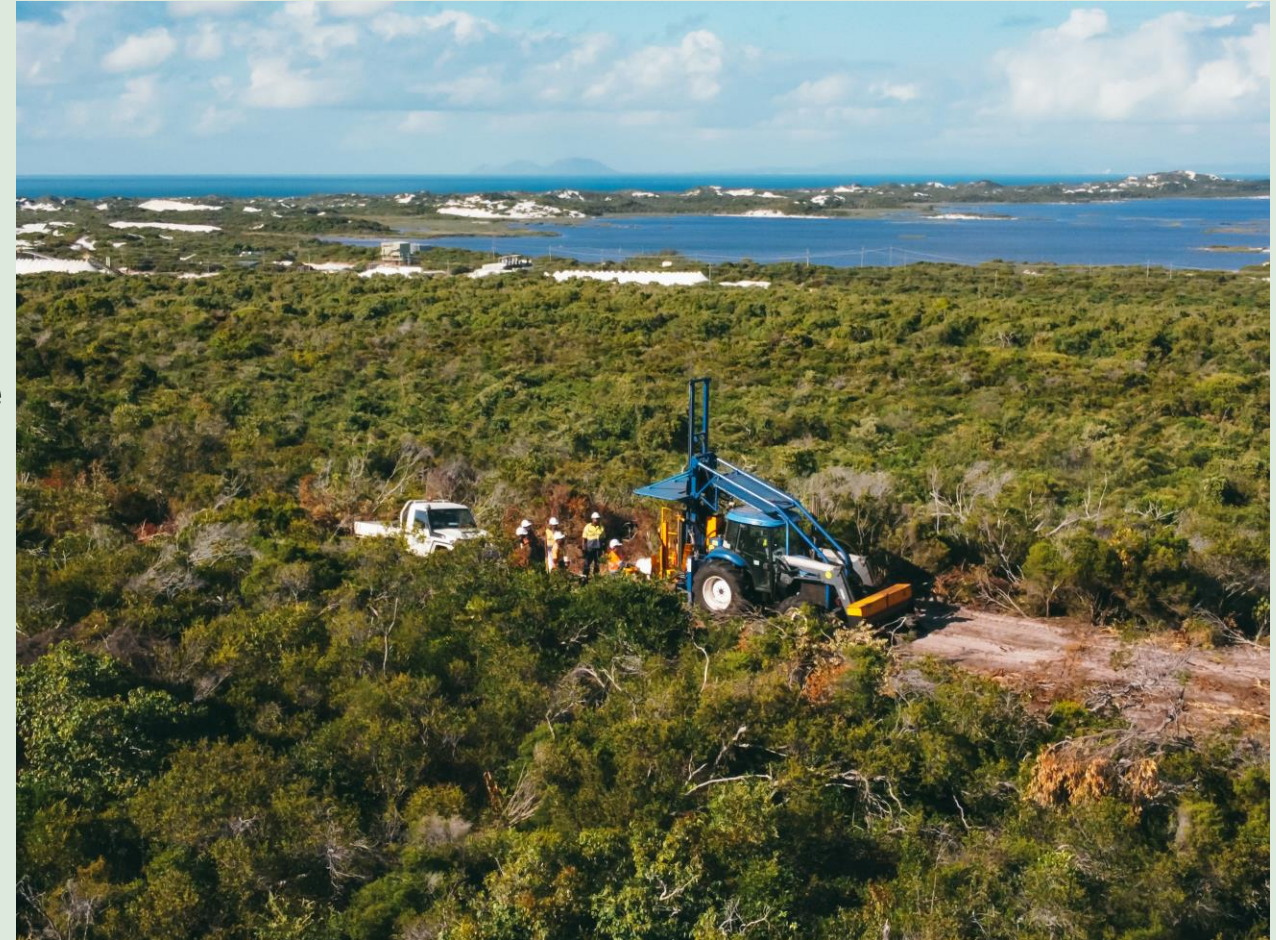
Cape Flattery drilling July/August 2021
