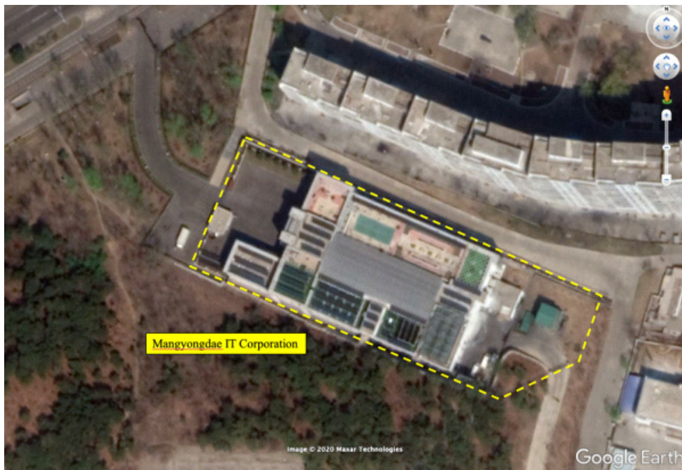
Figure 23. Mangyongdae IT Corp building in Pyongyang. (Image: Annotation by Martyn Williams /Google Earth)
