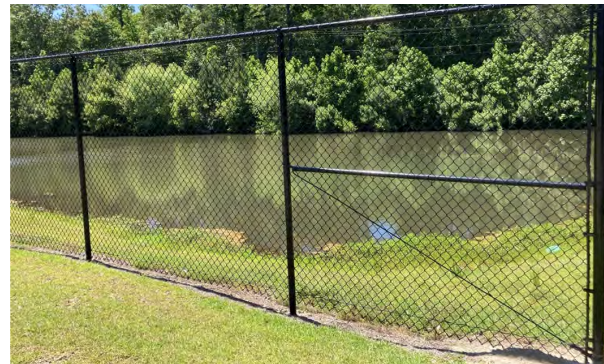
New exclusion fencing to dam
