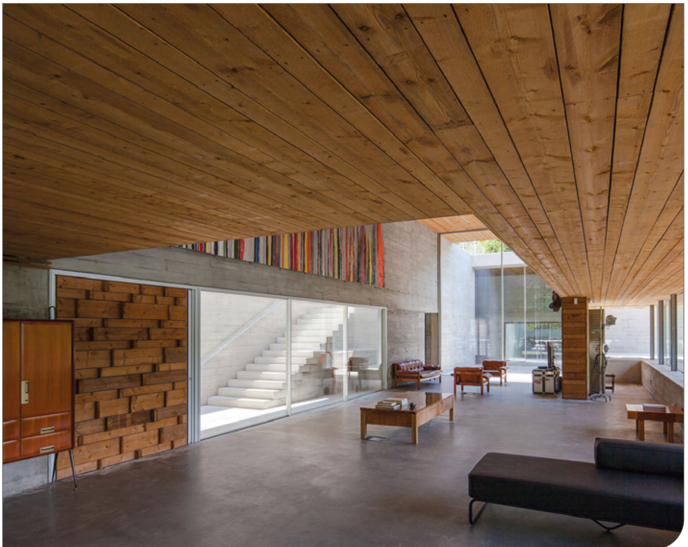
Figure 38. ThermoWood® ceiling in Portugal
