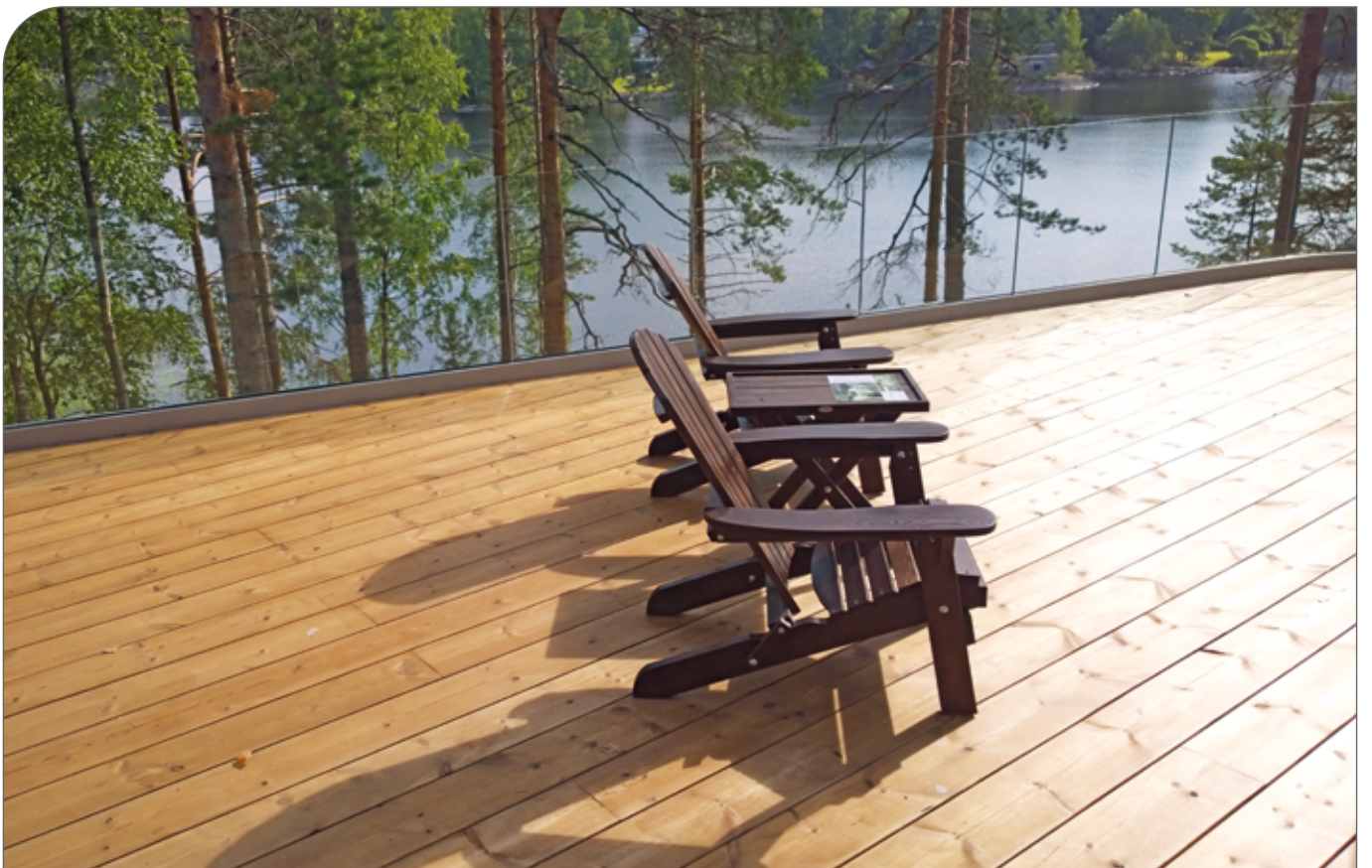
Figure 71. ThermoWood® terrace (Finland).
