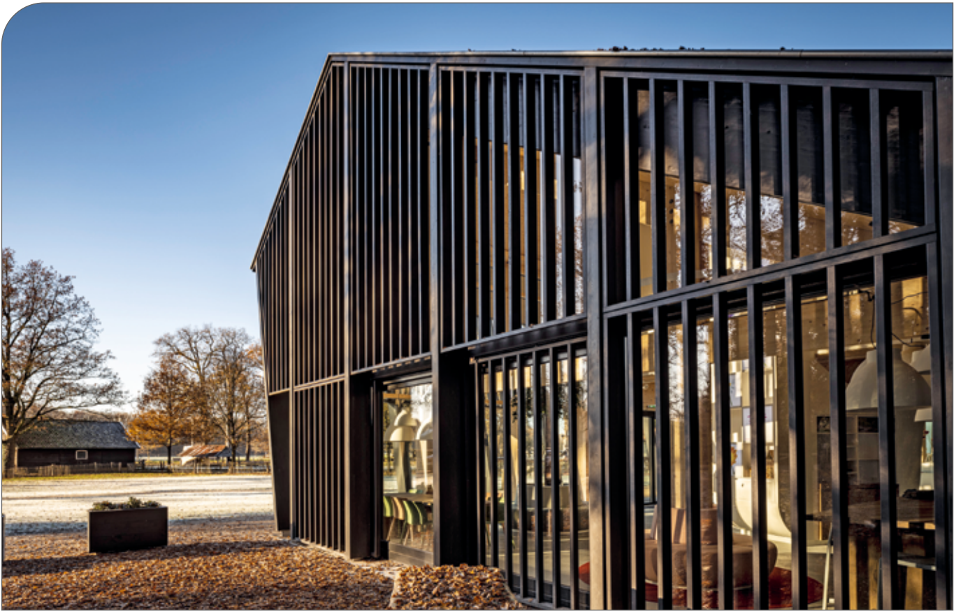
Figure 68. ThermoWood® exterior cladding (Netherlands).
