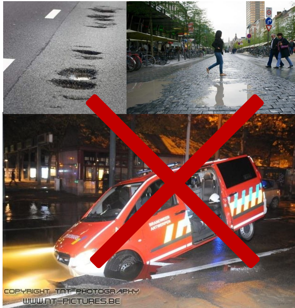
Discontinuities in pavement
