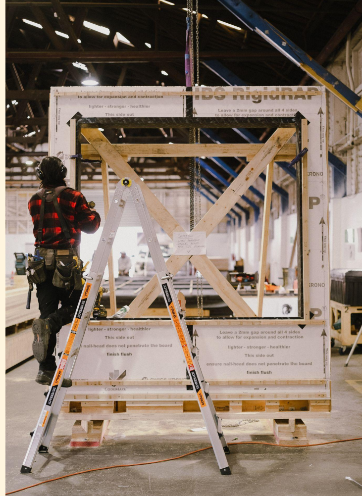
Flexi House Offsite Panel Construction
