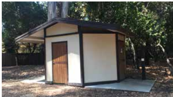
Porta-potty restroom structure
