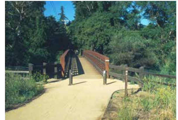
Bridge at creek
