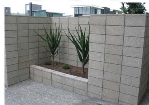
REFERENCE IMAGE CMU STACKED BOND WALL
