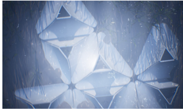
Fig 12. Blue Ceramics top view shows how sand is trapped
