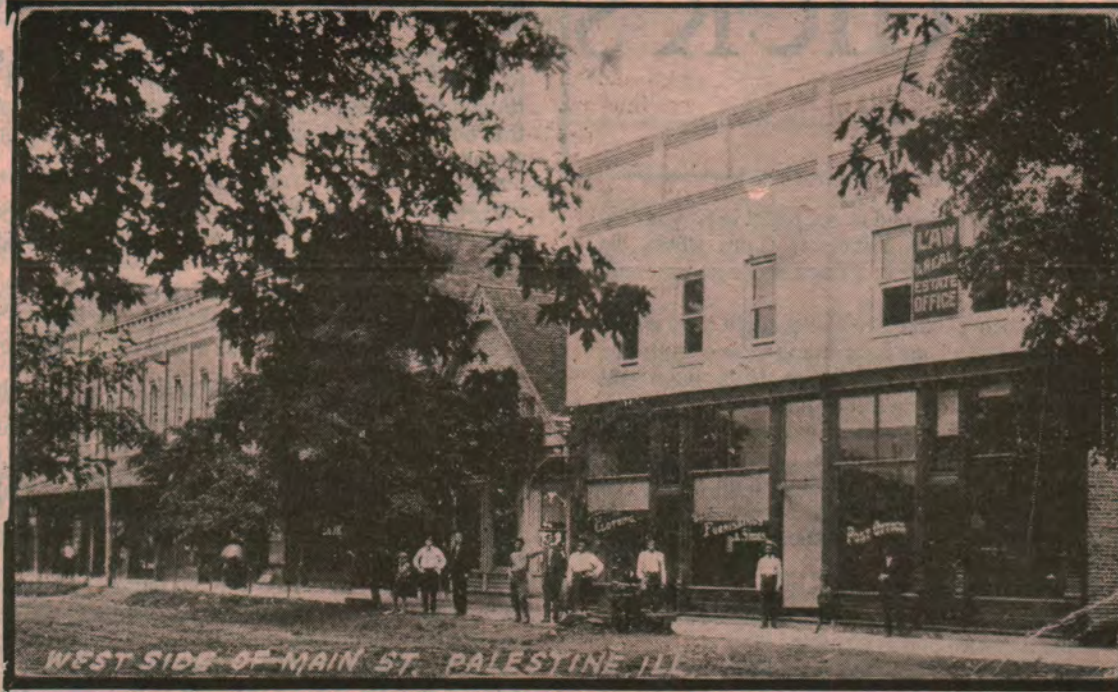
Postcard picture of the west side of Main Street in Palestine, Illinois, circa 1910.
