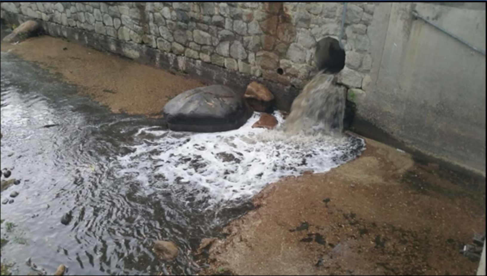
Stormwater discharge to the Truckee River from an urban outfall, City of Reno, Nevada
