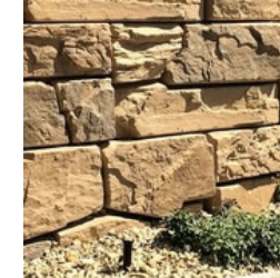
NATURAL STYLE BLOCK WALL
