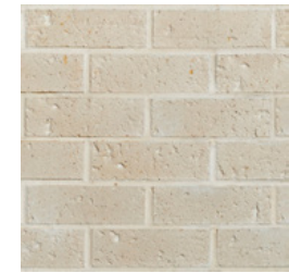
FACE BRICK FINISH
