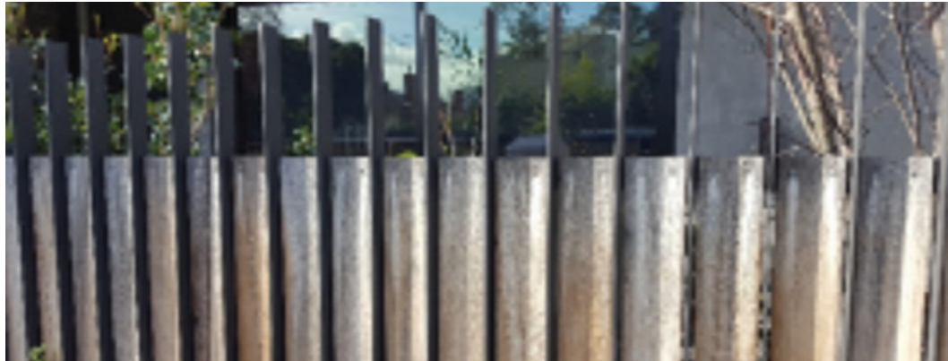
TYPE 4 : STEEL ANGLE PICKETS
