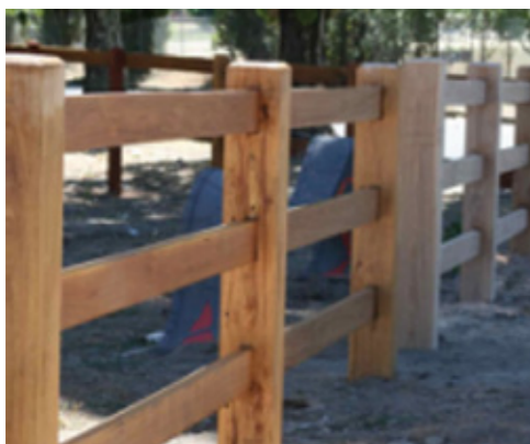
TYPE 6 : TIMBER POST AND RAIL
