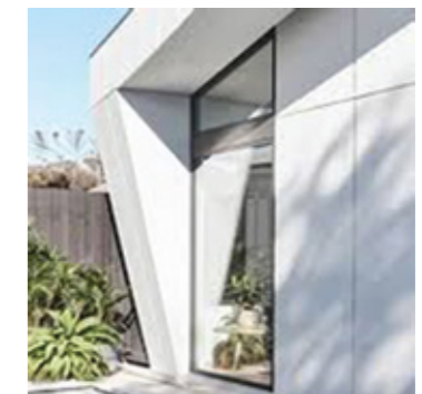
FC PRE-FINISHED CLADDING
