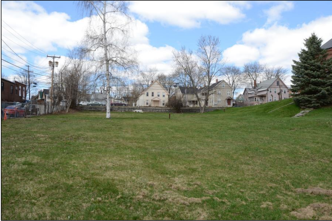
Photo 14. South Main Street retaining wall on the Concord Gas Light Co. parcel, looking west.
