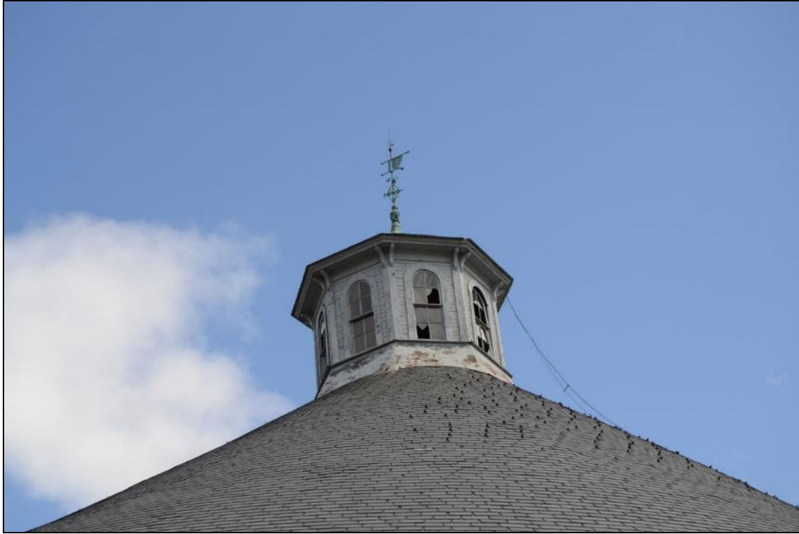
Photo 7. Detail of Gasholder House cupola, looking east.
