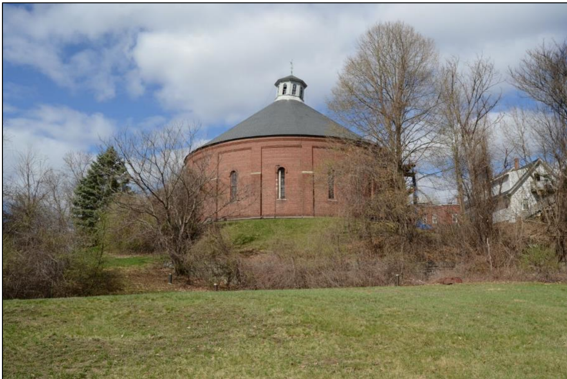
Photo 6. Gasholder House and its retaining wall, looking west from rear of Concord Gas Light Co. lot.
