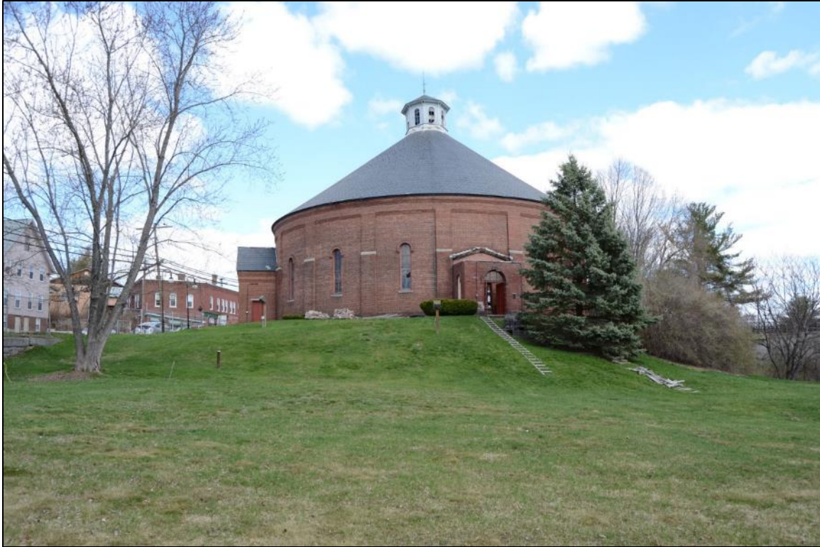
Photo 3. View of Gasholder House within Concord Gas Light Co. parcel, looking north.
