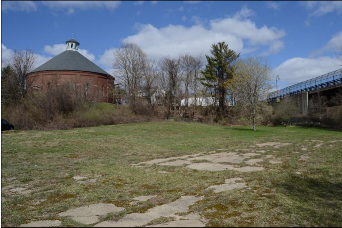
Photo 4. View of Gasholder House within former Concord Gas Light Co. parcel with foundation remains of gas plant and Water Street Bridge over former B&M RR tracks, looking northwest.
