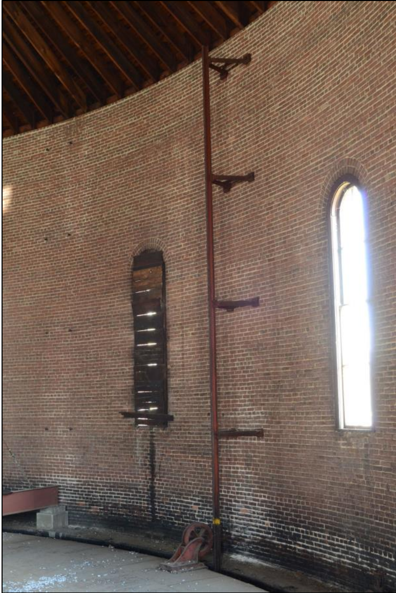
Photo 12. Detail of top of gasholder bell and gasholder guide, looking east.
