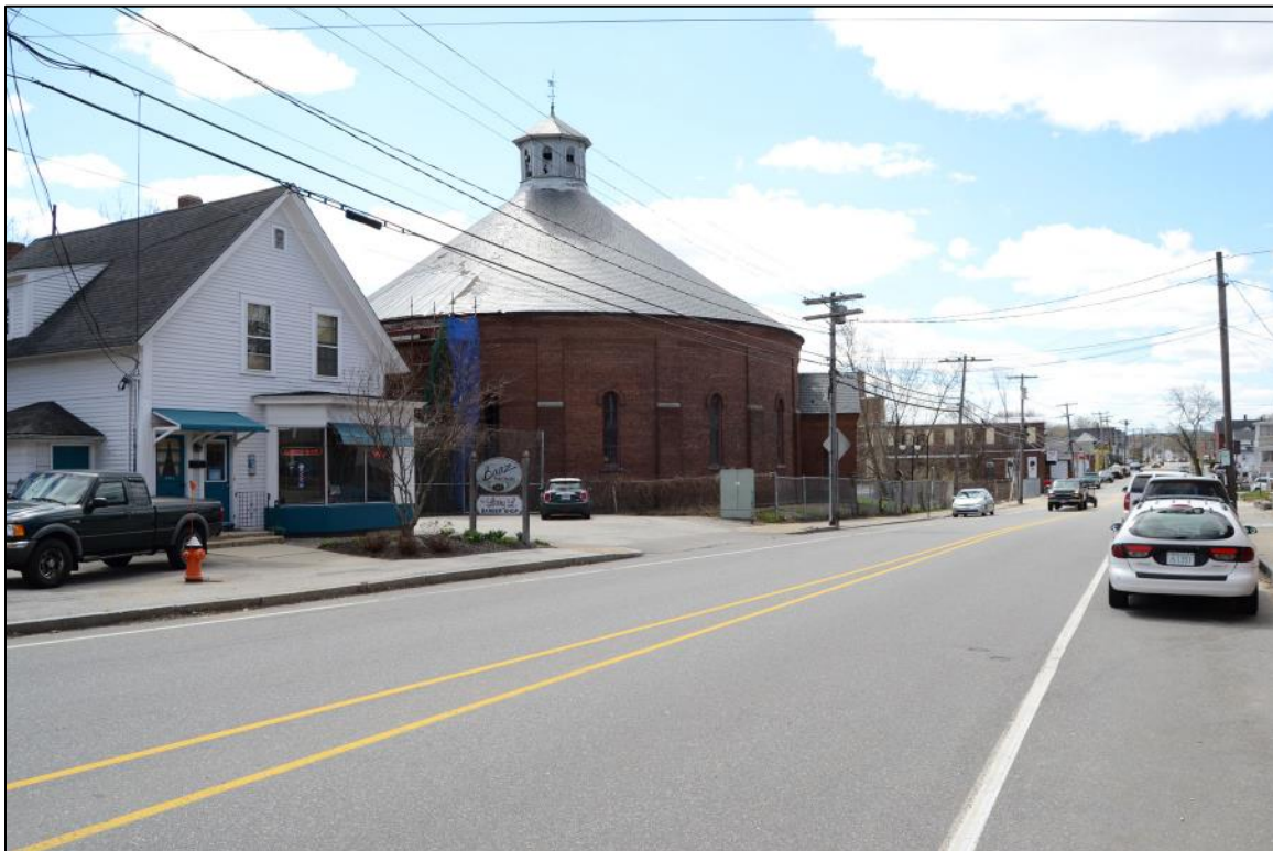
Photo 2. Gasholder House and its setting in the South Main Street manufacturing district, looking southeast from South Main Street.
