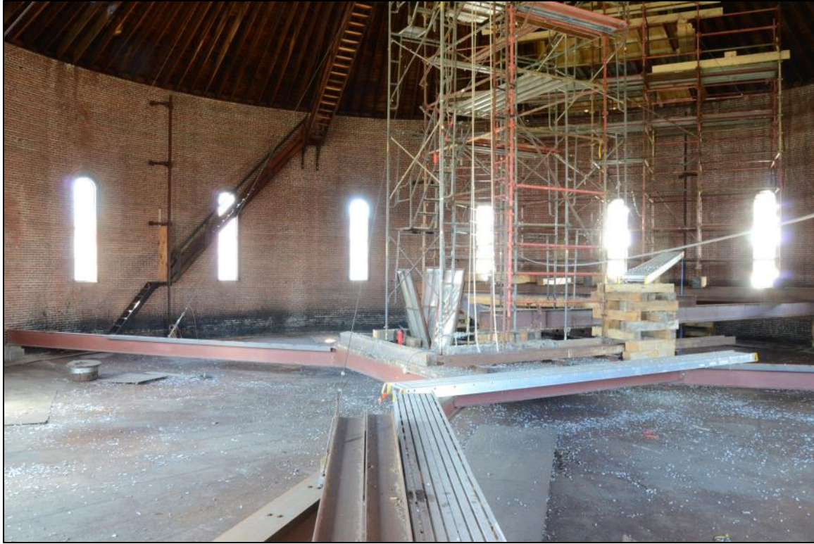
Photo 10. General view of Gasholder House interior showing top of gasholder's metal bell (the "floor"), looking north.
