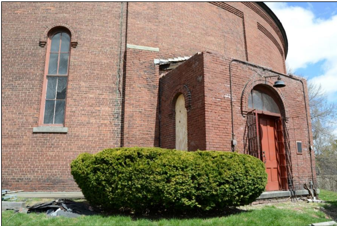
Photo 8. Detail of Gasholder House window and south valve house, looking northwest.
