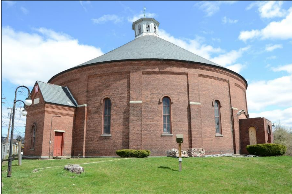
Photo 1. Concord Gas Light Co. Gasholder House (Gasholder House), looking northeast.
