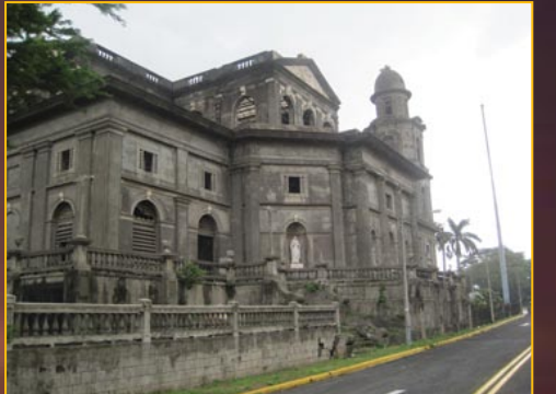
This is the Catholic Church in Managua, Nicaragua that was destroyed in an earthquake.
