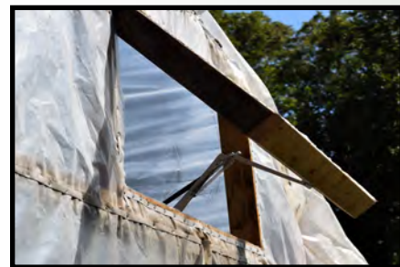
A farm-built automatic peak vent using a UniVent opener
