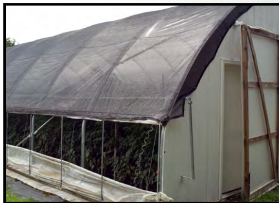
40% shade cloth installed on a high tunnel
