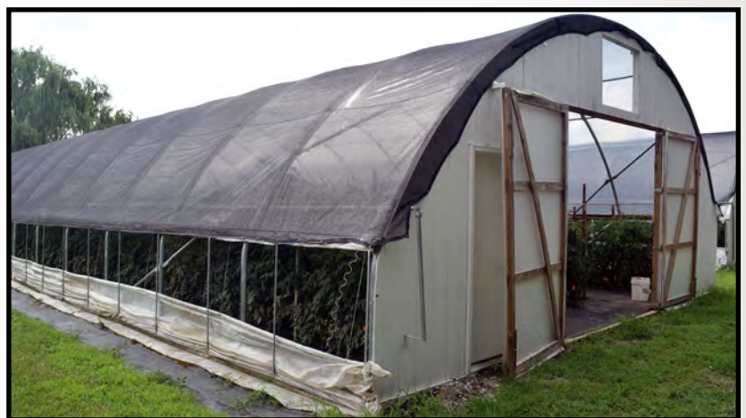
This tunnel at Gieringer's Orchard has a drop-down sidewall and open peak vent on the end wall.
