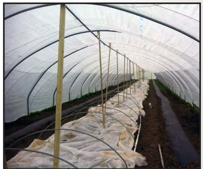
2' x 4' wood posts to hold bows in place on a three season high tunnel during a snow storm
