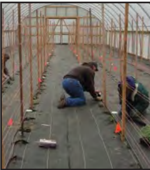
Laying landscape fabric and assembling the trellis system in a tunnel at Gieringer's Orchard during the winter
