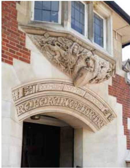
The restored entrance to Battersea Reference Library in Altenburg Gardens below left Inkwells become power outlets on the reading desks
