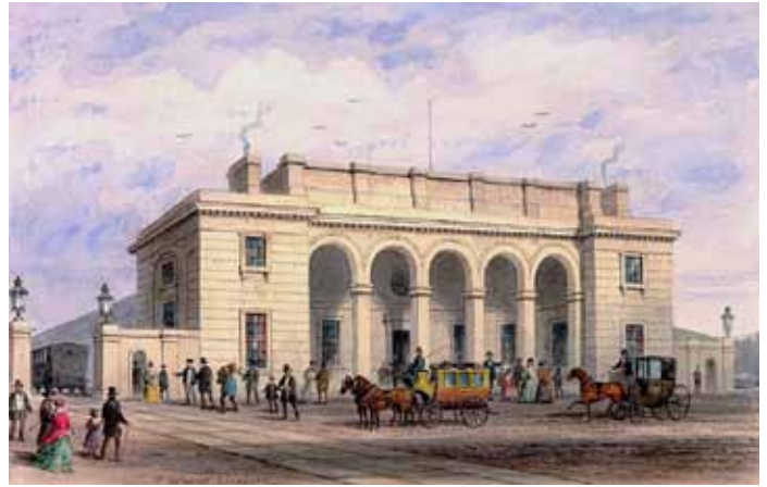
The neo-classical station at Nine Elms was designed by Sir William Tite, the architect of the Royal Exchange
