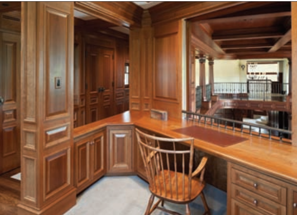
▼ WOOD PANELING , soffits with return grilles and crown mouldings highlight the second floor hallway.
