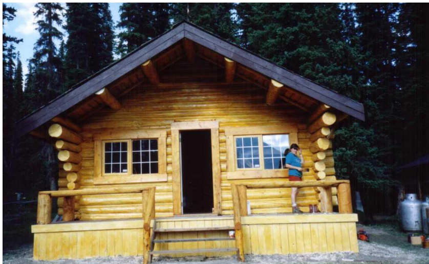
The original Shadow Lake cabin was transformed by major renovations in 1991.
