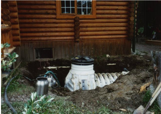
A new water holding tank was installed in 2000.
