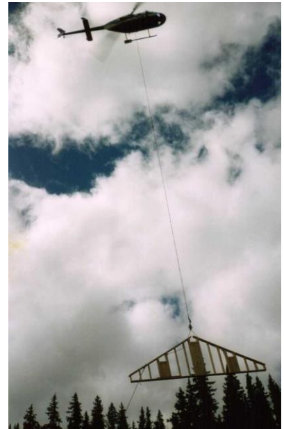
A helicopter slung the log purlons in place for the new dining cabin.
