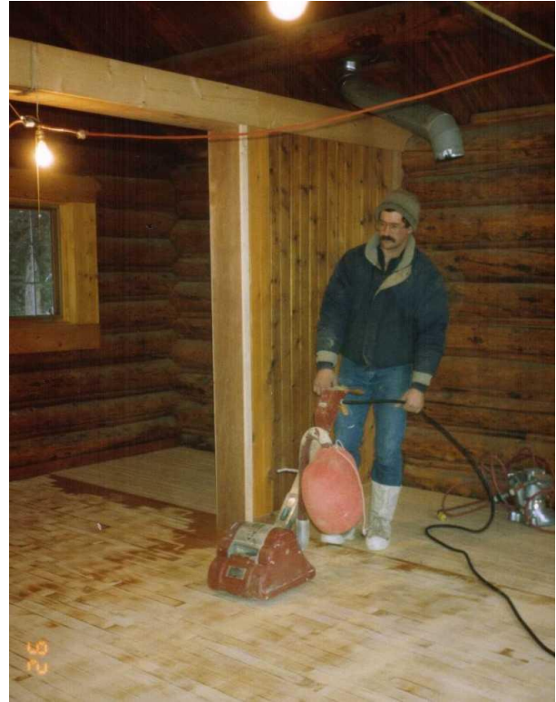
Bryan sanding the floor in preparation of opening, 1992.
