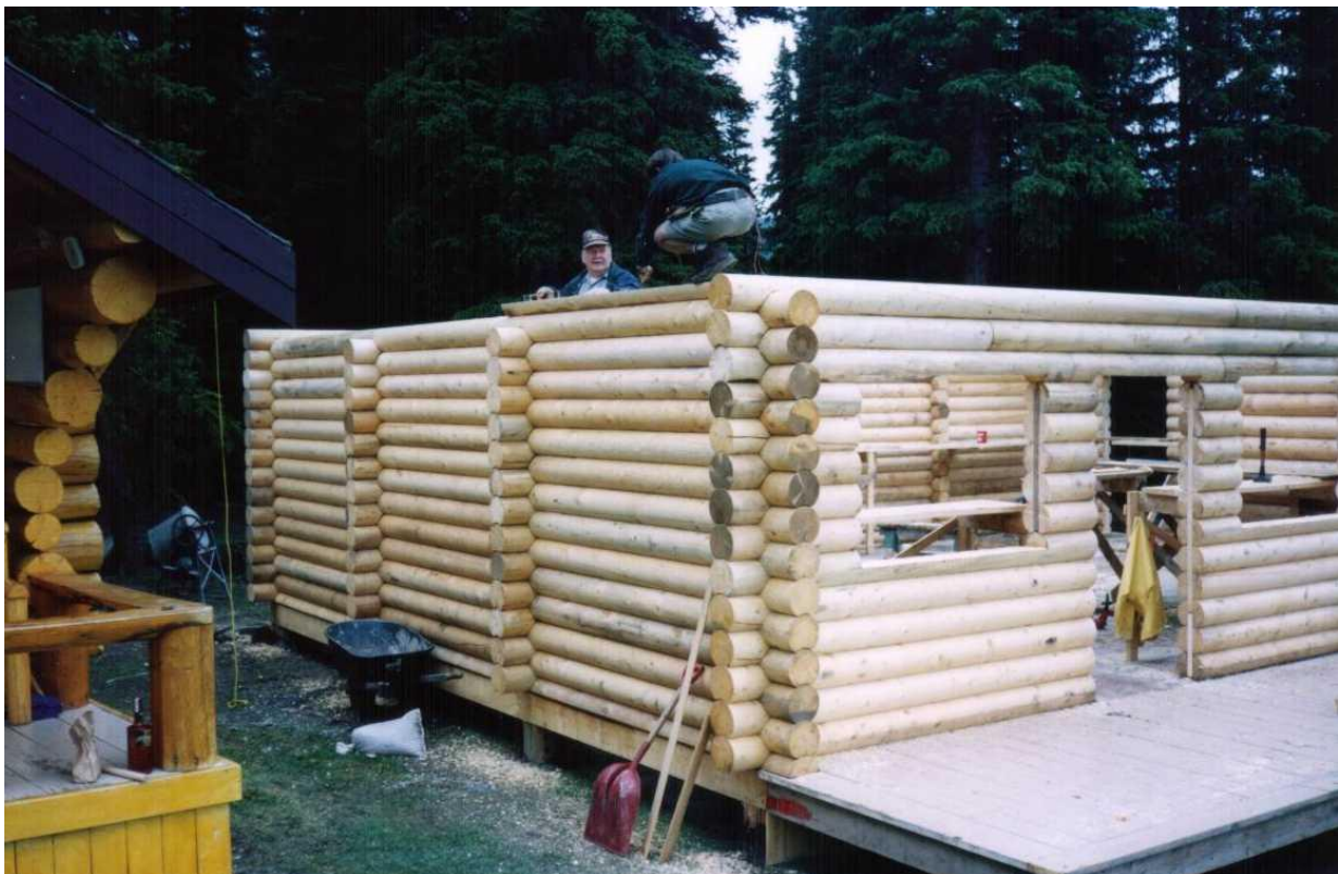
The new dining cabin takes shape, 1994.
