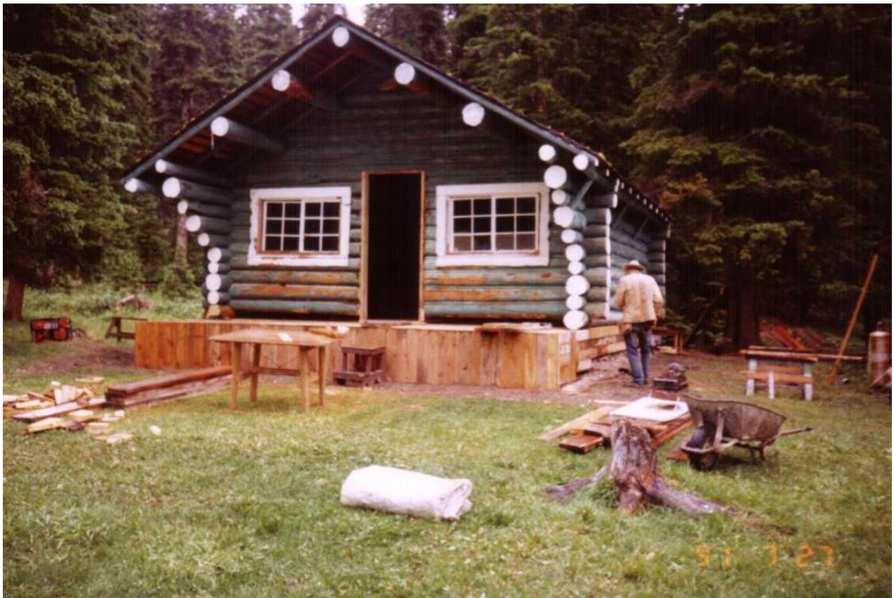
Renovations on the original cabin that took place in 1991 included adding a front porch.
