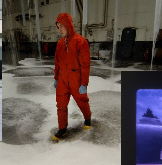
Fire Suppression Systems
