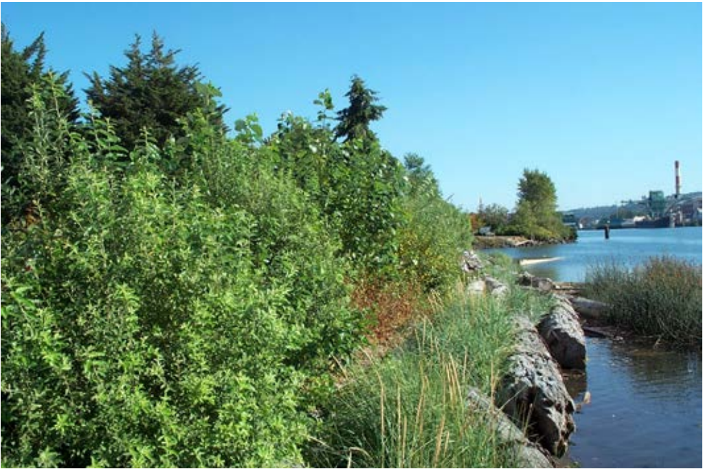
Figure #9: Soft Shore Stabilization Implementation at Terminal 108
